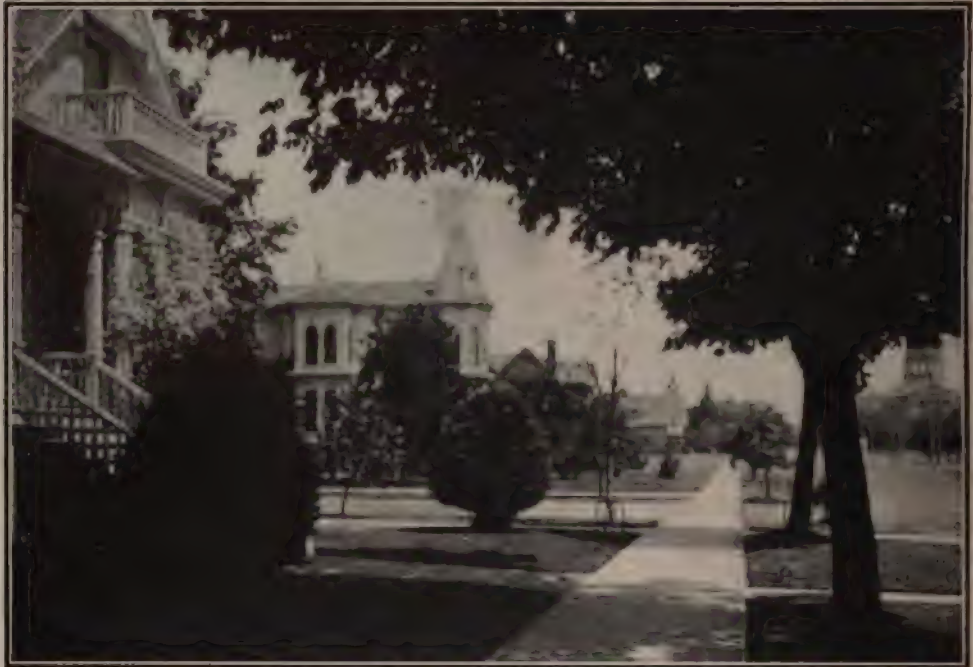
—the walk proper is from eight to twelve feet wide, leaving a strip from six to ten feet wide between the concrete and the street. This strip is planted with shrubbery, flowers and roses
